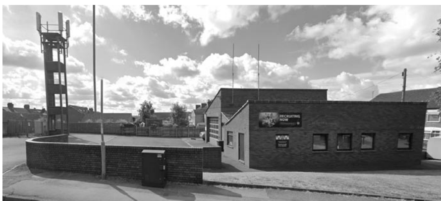
The on-call team at Desborough is moving to another station for about a month. The fire service says the condition of the station in Desborough, built in 1975, has deteriorated.
